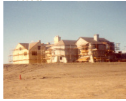
Construction of the winery
